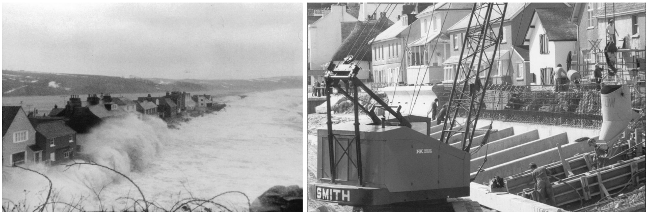
FIGURE 4. The sea wall at Torcross was built in 1979 after severe storms damaged houses. It is now being reinforced with double the depth of sheet piling in front of the existing wall (right).
