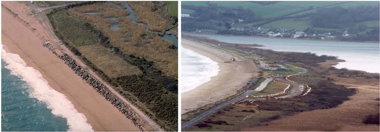
FIGURE 5. In 2001, storms undermined around 200 metres of the road along the Ley (left); it was 12 months before a new section was opened (right).
